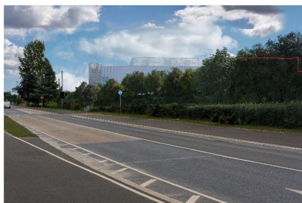
Figure 8-7N: Operation Stage Day 1: Viewpoint 6 – R134 New Nangor Road at the north west corner of the site looking south east.
